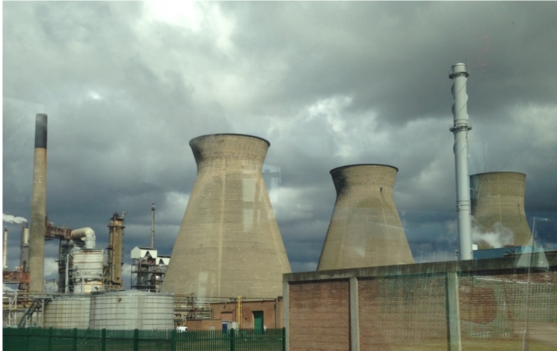
Figure 1. Cooling towers at Grangemouth industrial site.
